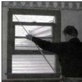
If the diagonals are not equal, it may be necessary to order a window 1/8" to 1/4" smaller than indicated by your measured height. This will allow the new window to be installed square in the opening. Then adequate sealing of the perimeter of the new window will complete the airtight installation.
